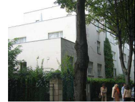
View street facade [Source: ERTL]
