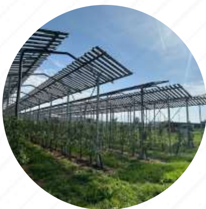
High construction installations (fruits) Orientation: eas-west
