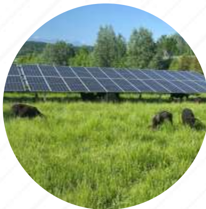
Low horizontal construction (pastures, permanent grassland) Orientation: South
