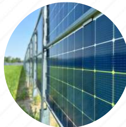
Vertical installation (cereals, vegetable, etc.) Orientation: eas-west
